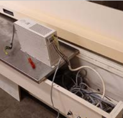
Paternoster's broken mains power supply filter.
